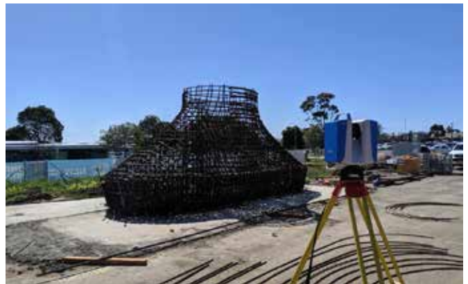
Scan of bridge headstock steel reinforcement cage to determine compliance to specifications. A heat map was used to illustrate non-conforming areas.
